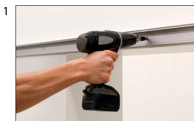
Fixing the track profile from the front
