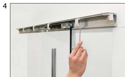
Fixing the clip covering holders with the same allen key
