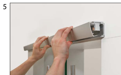
Clipping the covering profile into position
