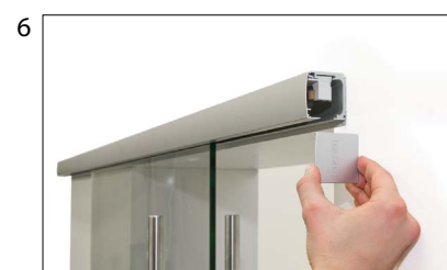
Attaching the end covers
